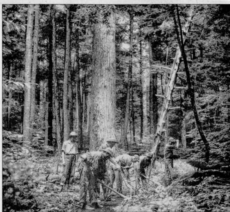
A Civilian Conservation Corps trail maintenance crew works in Nantahala National Forest in 1937. PHOTO COURTESY OF THE U.S. FOREST SERVICE
